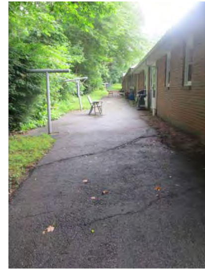
Asphalt-paved pedestrian walkways exhibit areas of cracks, tree root damage, and potential trip hazards
