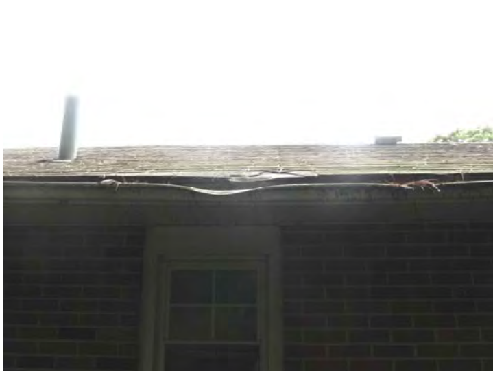
Gutters for roof drainage exhibit areas of damage at some locations
