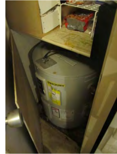
Each unit has its own, electric-type, domestic hot water tank
