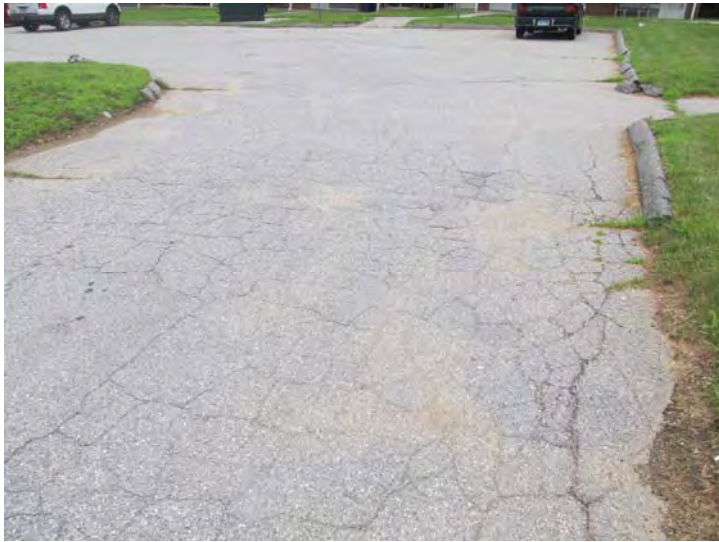
Asphalt paving at parking area exhibits age-related wear
