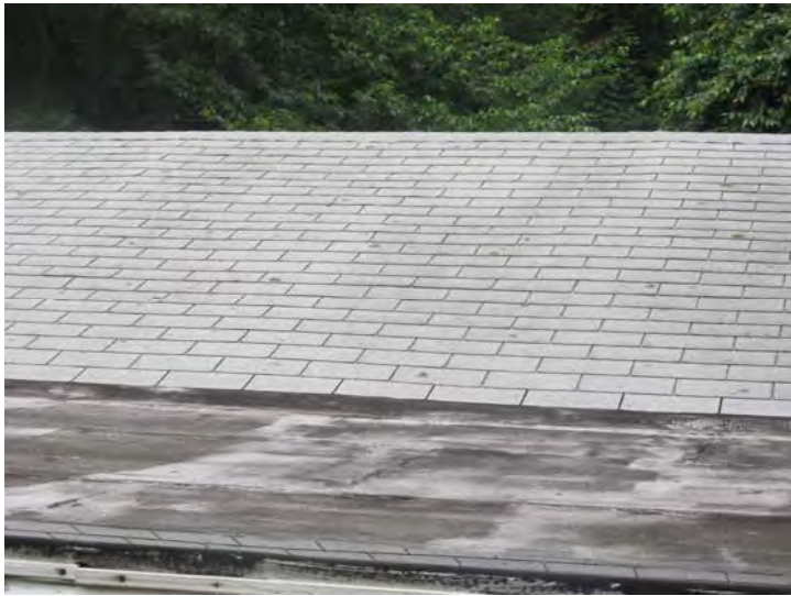
Older roof coverings that exhibit age-related wear are typical at all buildings
