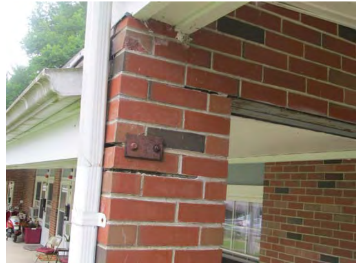
Isolated areas of mortar loss require repair/re-pointing
