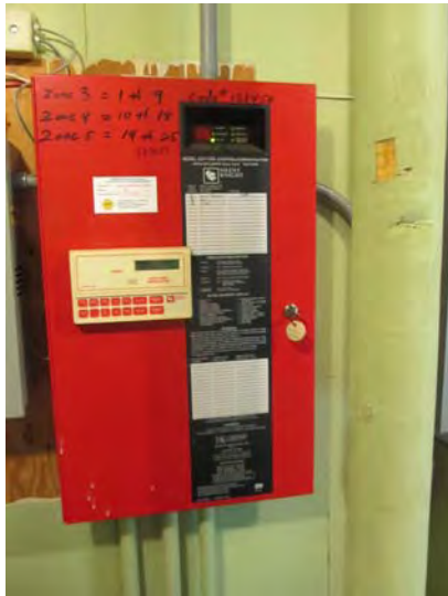
Fire alarm control panel monitors and supervises in-unit end devices
